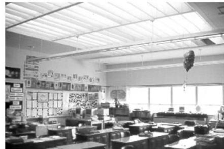
Figure 12—Seattle school with central skylight and diffusing louvers.
